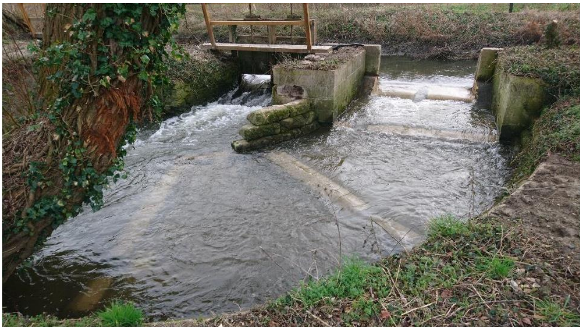
After: The weir height was lowered by approx. 250cm and gradient redistributed across a series of baffles. An alternate notch sequence was cut into the baffles and weir to manage flow speeds and ensure fish passage during low flows.
