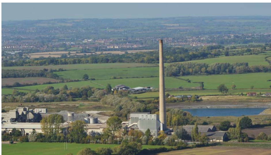
Westbury cement works. Photo: Paul McRae WWT
